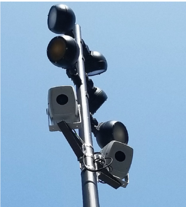
Atop a pair of 35-foot poles rising above Dilworth Park are box-like fixtures at the lower end of the pole containing additional LED fixtures that project color lighting onto the columns of mist, amplifying and diversifying the hues projected from beneath the surface grating.
